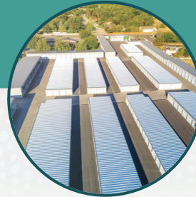
Expansion of an existing facility
