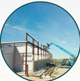
Ground up Construction
